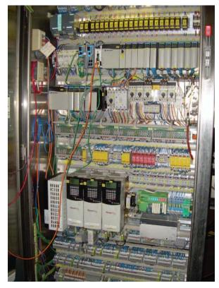
This automation cabinet contains power, control, and communication wiring. A 480-volt disconnect handle is at the upper right of the cabinet. PLCs near the top of the cabinet use 24-volt inputs and outputs to control a conveyor system while 480-volt VFDs near the cabinet bottom drive the conveyor motors.
